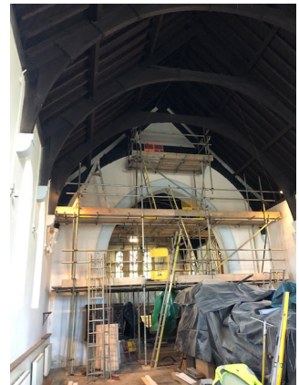
Shows painting the Chancel new radiators, spot lights and Wainscoting.
