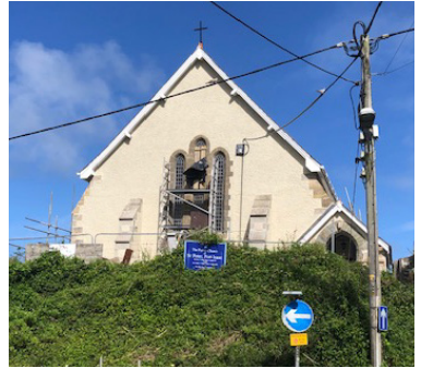
New colour of outside. Scaffolding is now down
